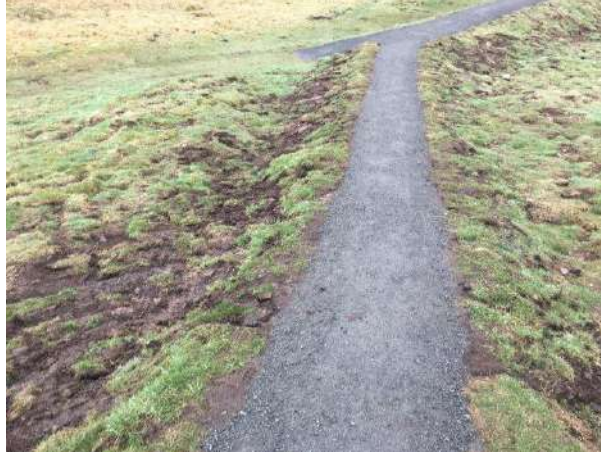
14.2 Some impacts on reinstatement on Dumyat from cattle.
