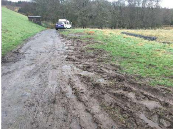
14.1 Disturbed ground at eastern end of reservoir.
