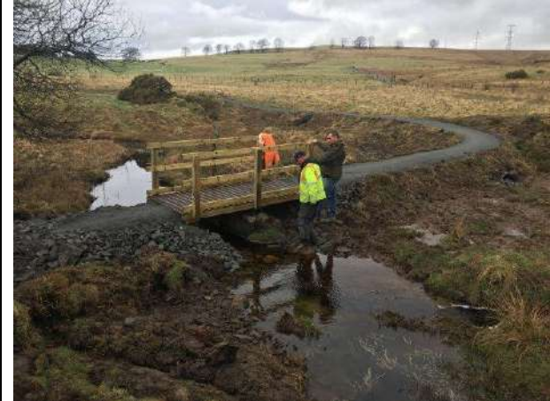
Bridge installation complete including high flow side channel.
