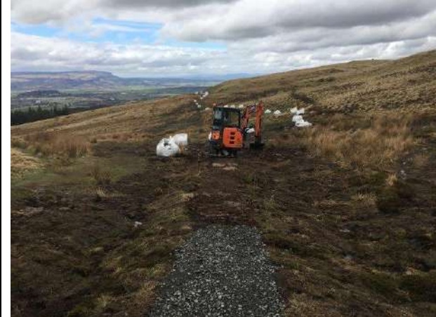
14.3 Start of Section 6 under construction.
