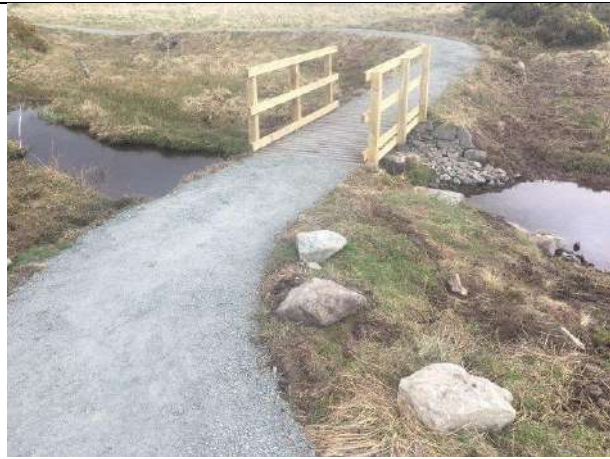
Bridge installation and good reinstatement
