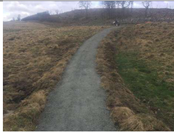
11.1 Section cleared of material and reinstated
