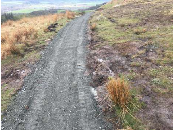
16.5 Section of wet ground that requires drainage management.
