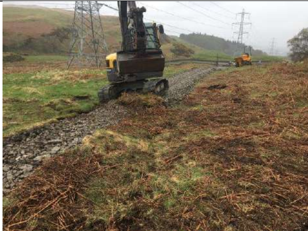
Continuation of good reinstatement along Cocksburn.
