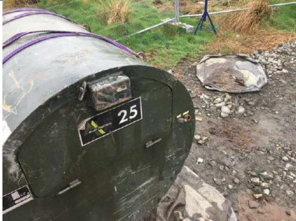
16.1 Fuel bowser not locked and unattended.
